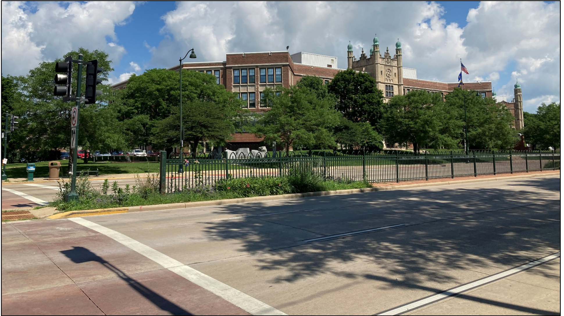
Figure 41. E. Washington Avenue at 4 th Street, View North – Existing Madison East High School in Background
