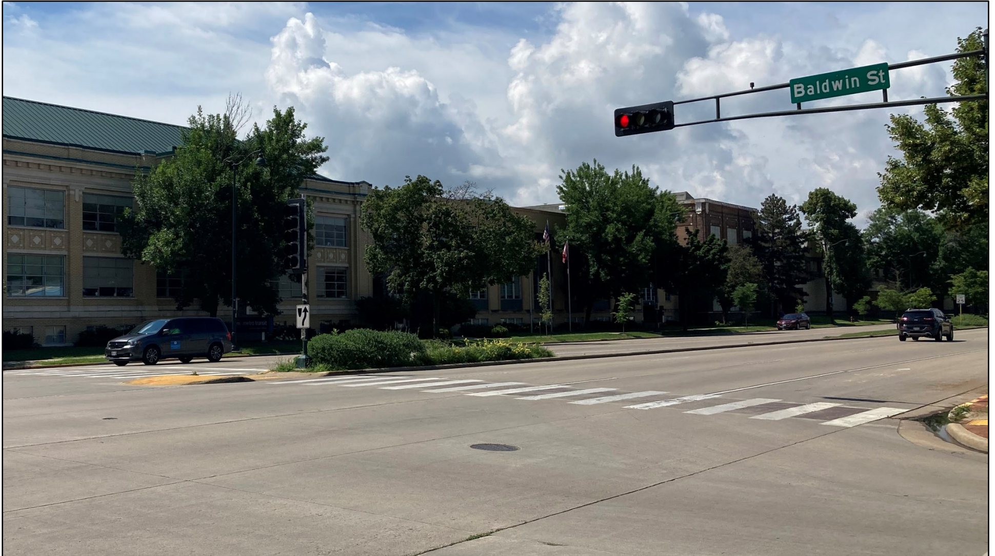
Figure 38. E. Washington Avenue at Baldwin Street, View South – Existing Gisholt Machine Company in Background
